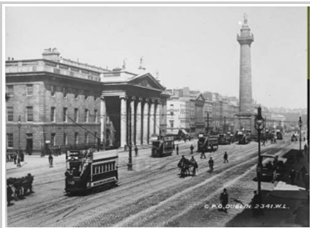
Sackville Street. Courtesy: National Library of Ireland.
